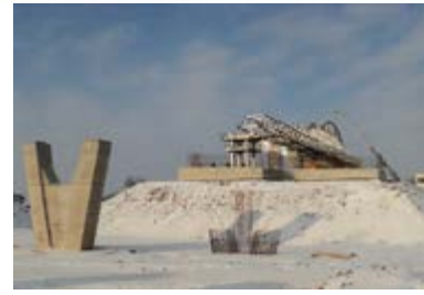
Opatovický Canal Current Span 42 m Czech Rep.
