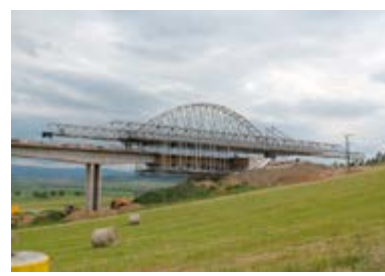
Viadcut J216 – Janovce Current Span: 65 m Slovakia
