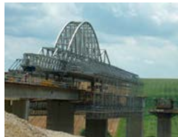
Viaduct J17 Jablonov, Current Span: 65 m Slovakia
