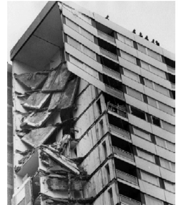
Ronan Point apartment building progressive collapse, 16th may 1968.
