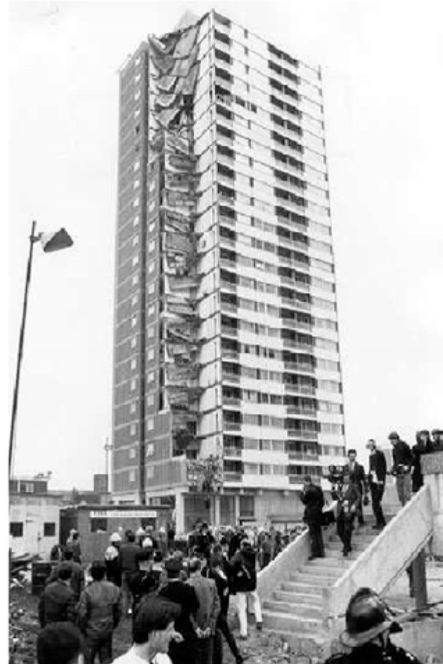
Ronan Point apartment building progressive collapse, 16th may 1968.
