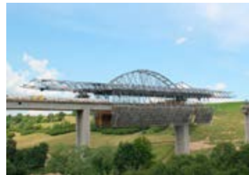
Viaduct SO202 Fricovce Current Span: 45 m Slovakia
