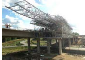
Viaduct ins Sokolov-Tisova Current Span: 42 m Czech Rep.
