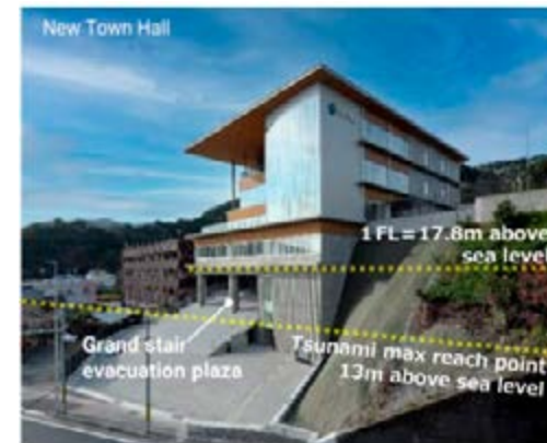
Open space for evacuation planned above the predicted flood height = T.P13m
